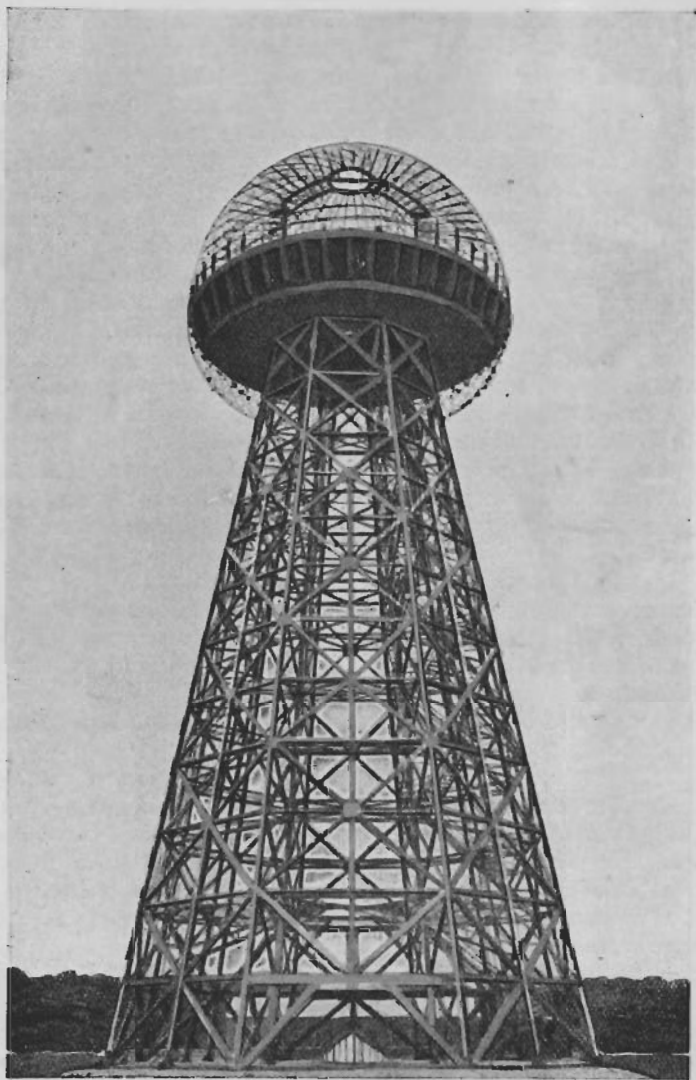
FIG. 136.—MR TESLA'S TRANSMITTING STATION ON LONG ISLAND.
